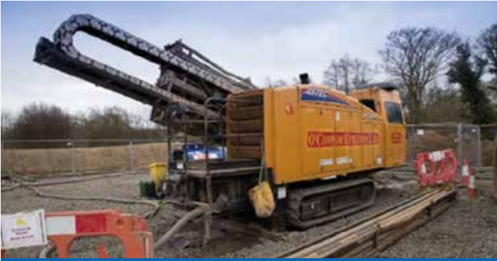
Example Horizontal Directional Drilling (HDD) Rig
